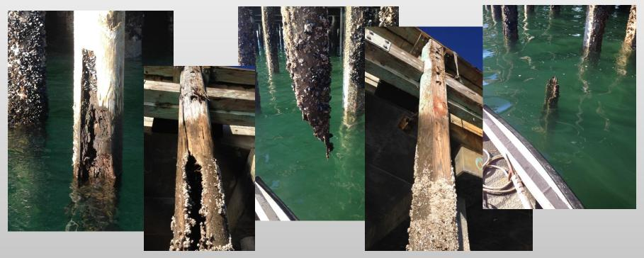
Current treated timber system heavily deteriorated and at the end of its service life
